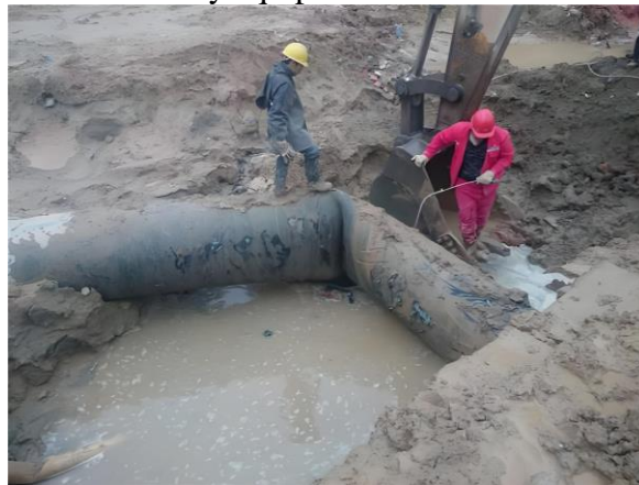
Figure 2. Oil leakage caused by aging of oil pipelines
